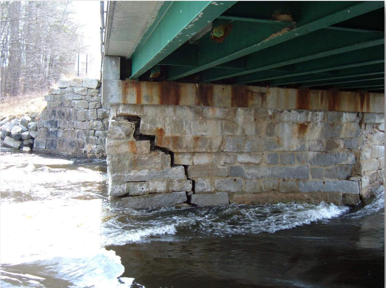
Damage to Lee Hook Road, Flooding
